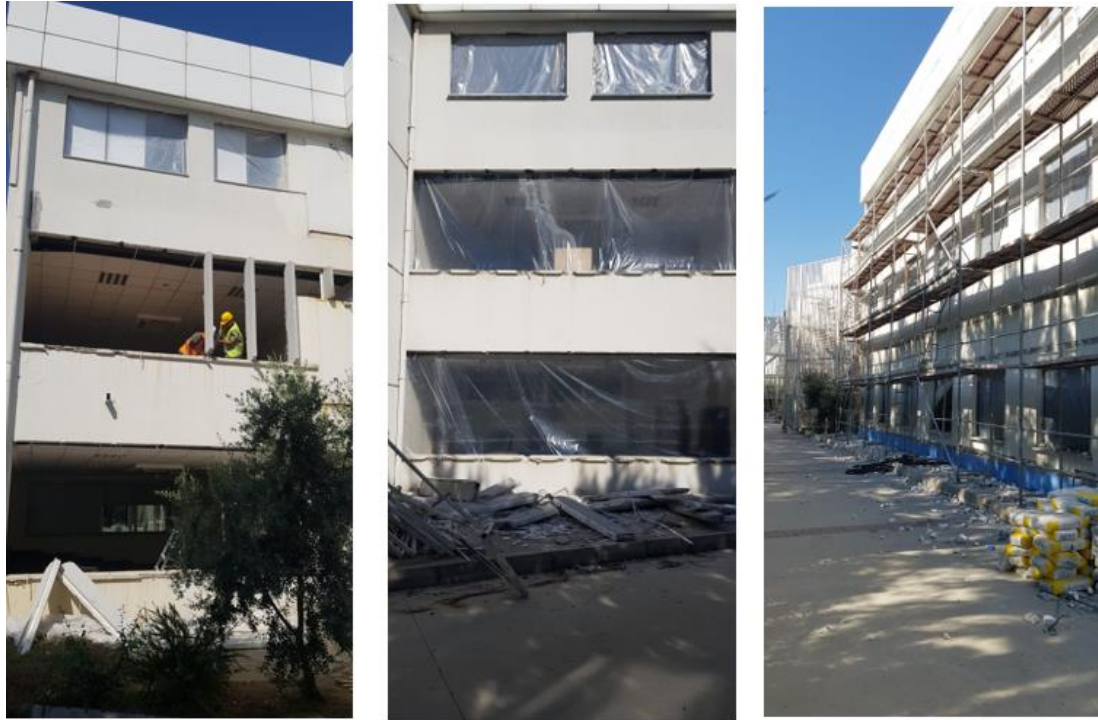
Figure 11: Facade insulation and window replacement at Izmir Bakircay University (August 2023)
